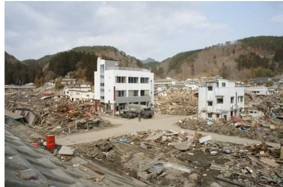
Figure 4. Buildings which survived during the tsunami in Taro area
