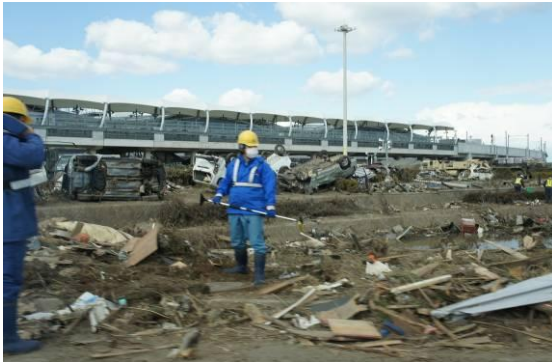
Figure 23. Damages around the airport
