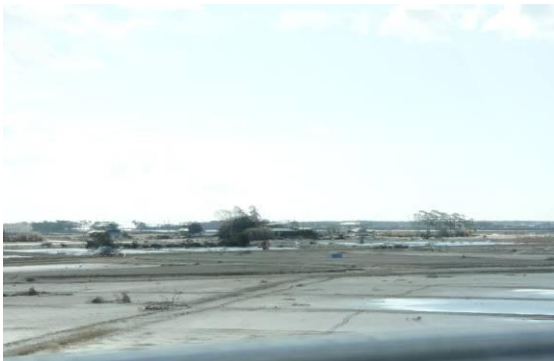
Figure 16. Damages by the tsunami
