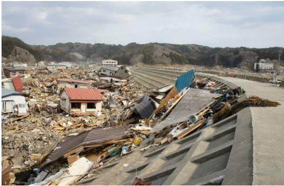
Figure 3. Damages by the tsunami in Taro area
