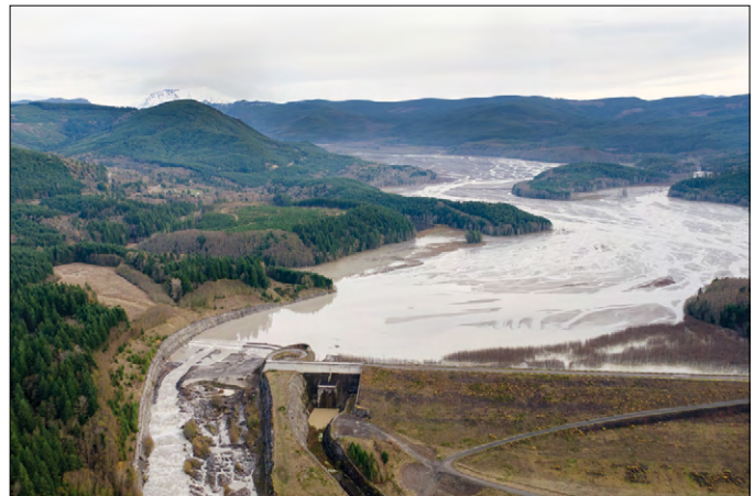
Figure 30. Photograph of the 575-meter-wide sediment retention structure (SRS) on the North Fork Toutle River. The structure is located 35 kilometers downstream from Mount St. Helens, which is visible in the background, in the North Fork Toutle River basin. The SRS was designed to trap nearly 200 million cubic meters of sediment and nearly reached capacity by 2012, after which the spillway was raised slightly to extend the lifespan of the sediment trap. USGS photograph by A.R. Mosbrucker, 2012.
