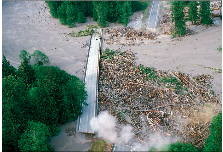
Figure 27. Aerial photographic view of the North Fork Toutle River lahar on the afternoon of May 18, 1980. This photograph was taken at the moment the lahar pushed the State Route 504 bridge off its support piers. The location is just downstream of the North and South Fork Toutle River confluence. The bridge deck was never found. Photograph by Roger Werth, The Daily News (Longview, Wash.), copyright 1980.
