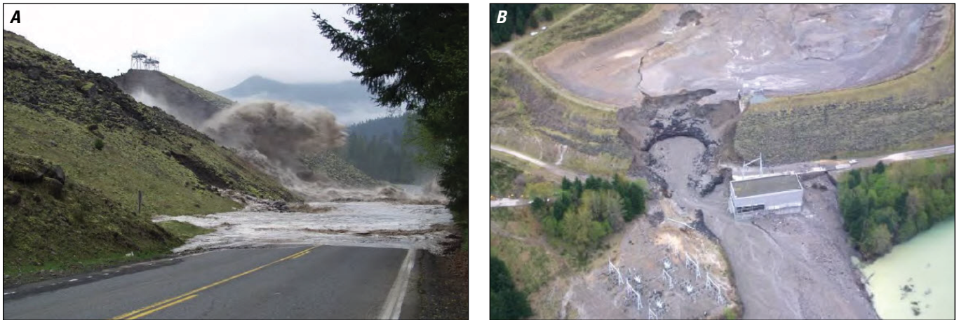
Figure 47. Failure of the Swift Reservoir power canal dam. A. Photograph showing the blowout of the power canal dam and flooding of Forest Road 90 at about 6:55 a.m. on April 21, 2002. PacifiCorp photograph by T. Low, 2002. B. Aerial photograph of dam failure and the damage to power-generating facility. Note the sinkhole into the Cave Basalt lava flow at top center of frame. USGS photograph by C.D. Miller, 2002.
